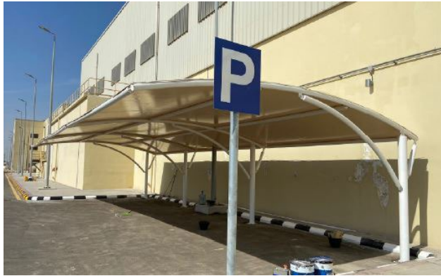
Carpark Shed Plant-1
